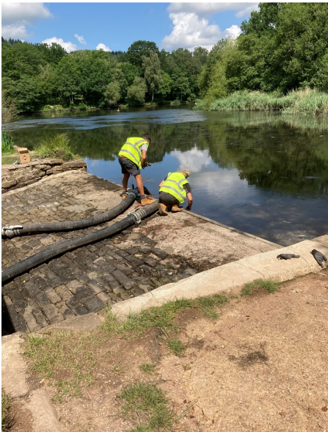
Contractor refurbishing weir?
