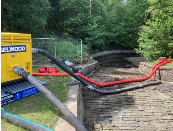
A huge pump took water from one side of the spillway to the other
