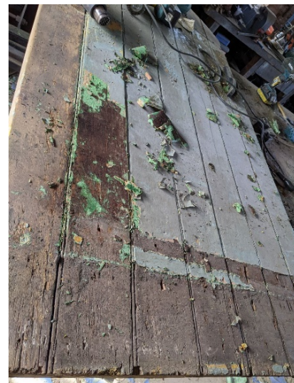
Paint being stripped off
