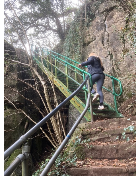
The metal staircase close to the top
